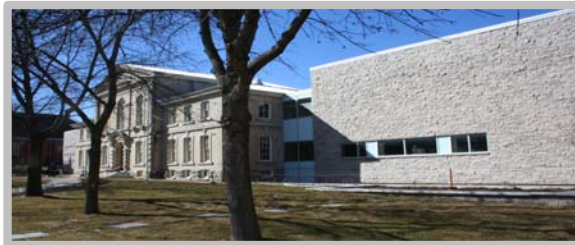
After renovation and restoration (2007)
